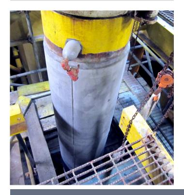
Nautec provided the strengthening method to repair corroded surface casings of well heads at a platform offshore Sarawak. Upon the visual inspection of one of Shell's platforms, 2 wells were found to be corroded and immediate measures were taken to arrest further corrosion and repair the damaged areas of the well conductors and structural casings of the platform.
