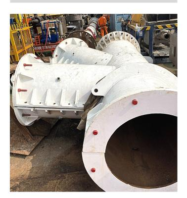
In December 2021, Nautec carried out Horizontal Member repair services for Larsen & Toubro Hydrocarbon Engineering Limited using Nautec's proprietary NaX<sup>®</sup> Q140-E UHPC grout.
