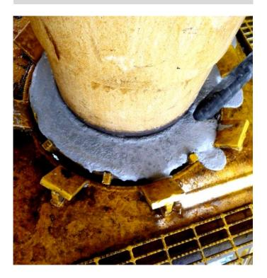
Well inspections carried out by Brunei Shell Petroleum revealed that a significant number of wells were suffering from acute corrosion.
