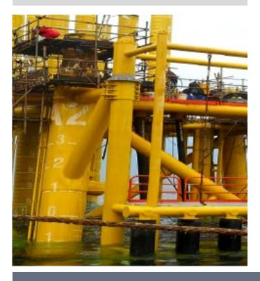
Provision of grouting services for SA-SA Jacket Installation. Grouting of Jacket Leg Annulus.
