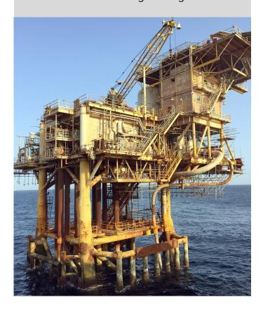
Nautec has completed the underwater strengthening work for 2 platforms as part of C-26 Cluster Pipeline Project for SWIBER in India.
